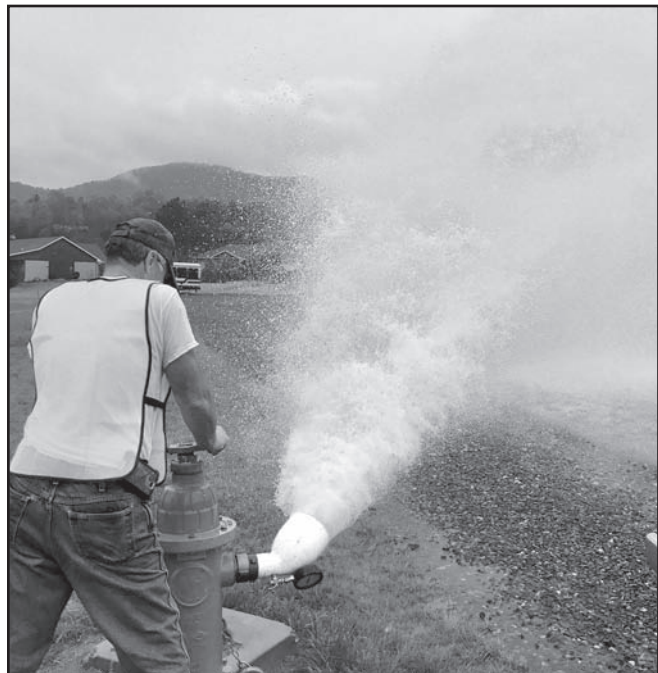
The City of Hiawassee flushed its 201 hydrants last month between April 18 and April 20.
